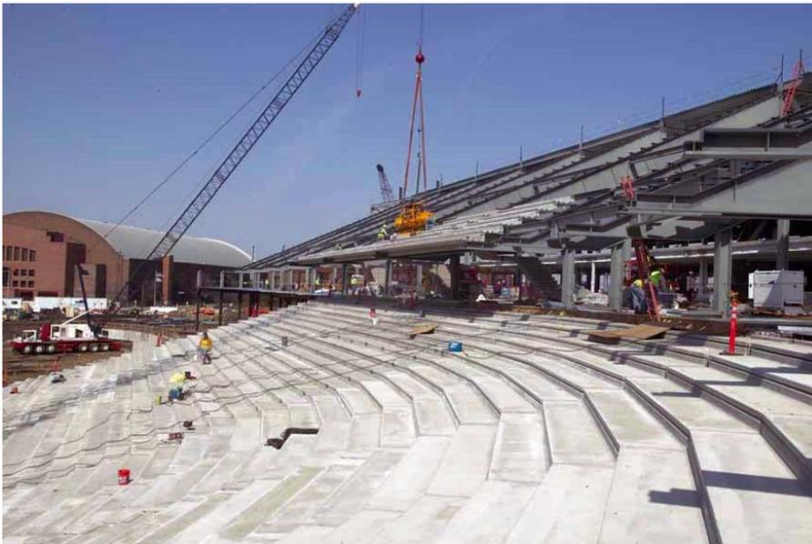
*Thanks to the vacuum handling devices, Hanson was able to cast the units with no inserts on either side for conventional lifting*
