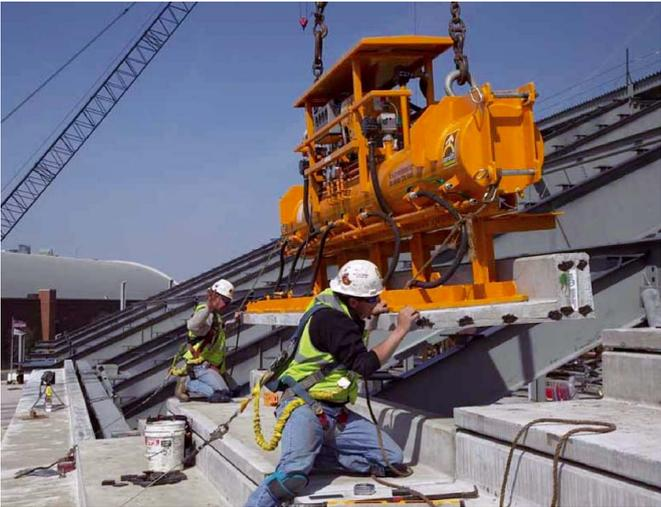
Vakuum lifting devices provide an optimal handling solution of pre-cast concrete
