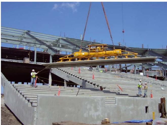
*Concrete cast with no inserts on either side as with conventional lifting*
